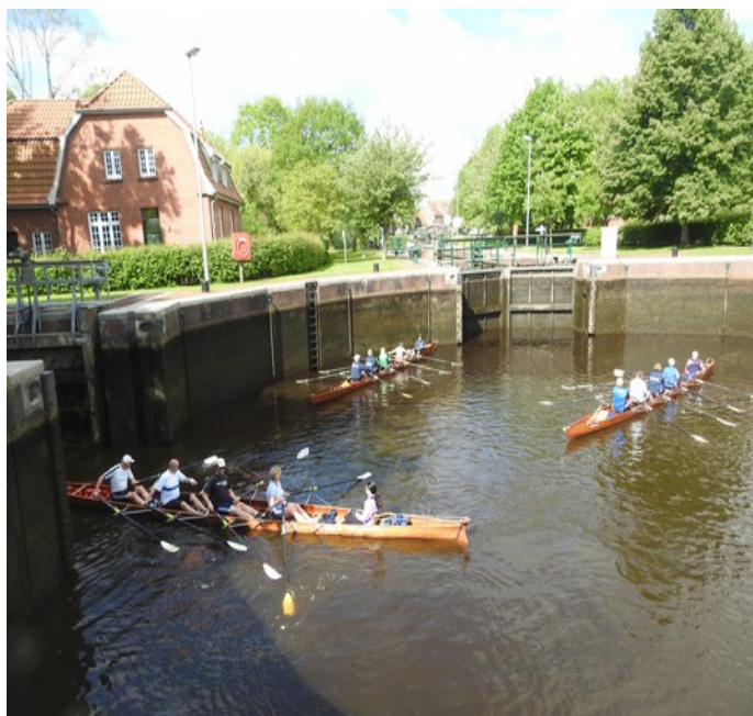
Kesselschleuse in Emden
